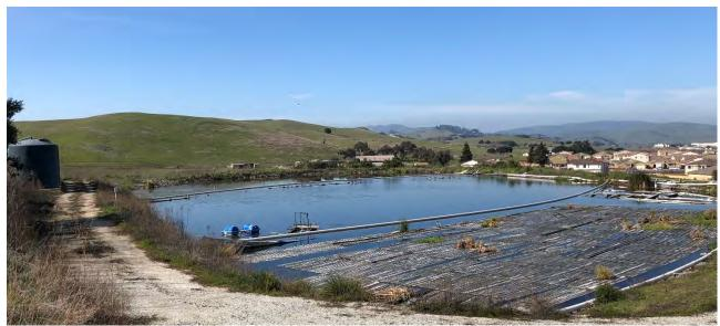
Figure 12 is a picture of Pond 2, including the sludge storage lagoon and polishing pond.
